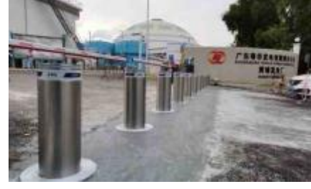
Guangdong Yuehua Power Plant
