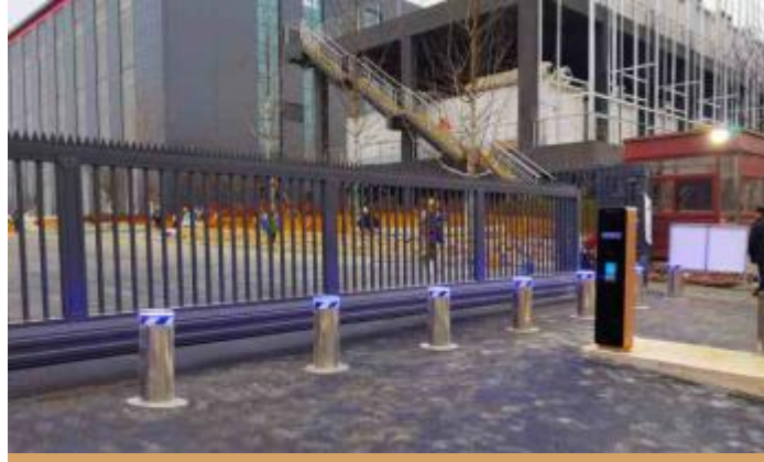
Huawei Cloud Data Center
